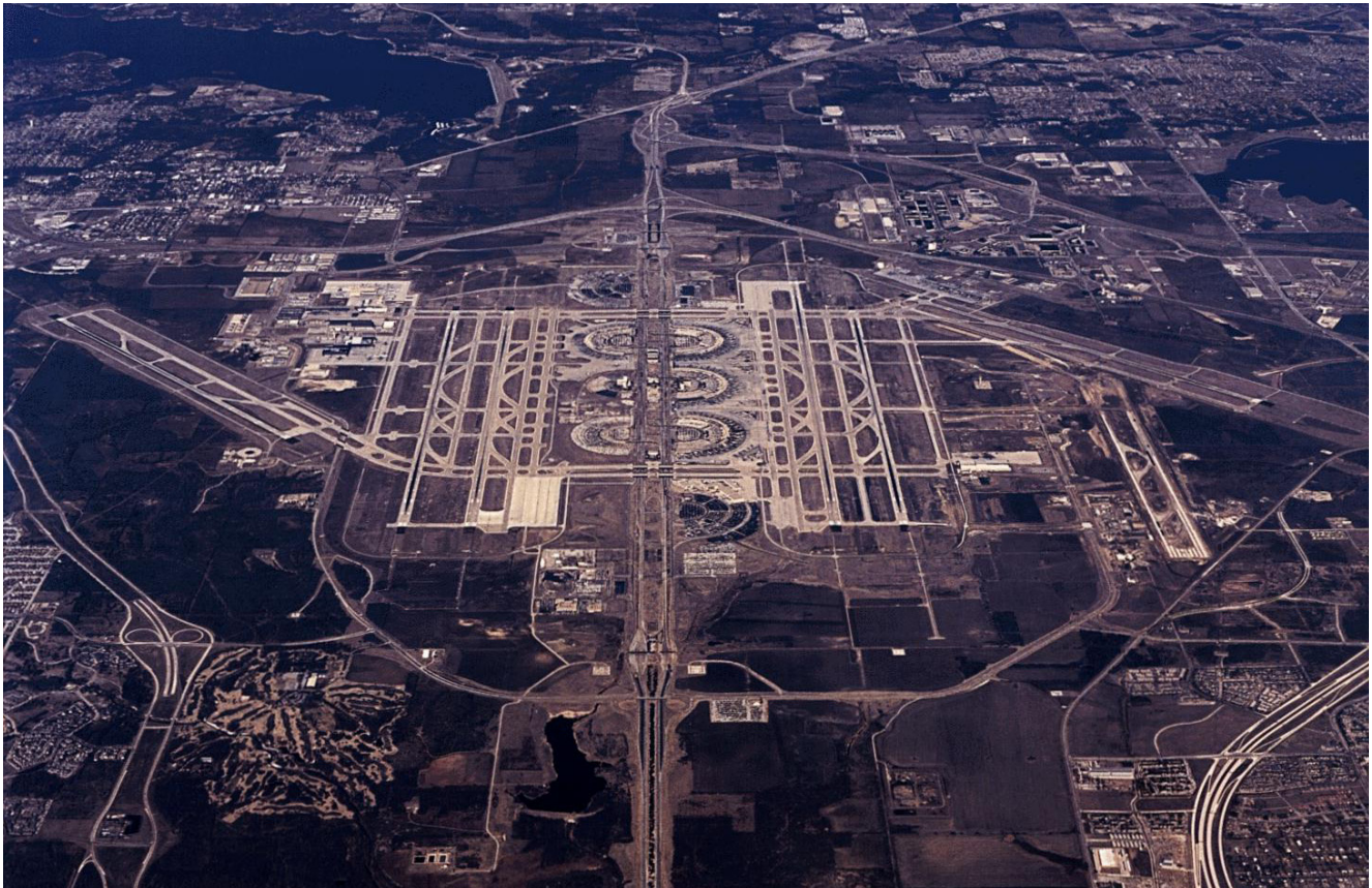
Dallas/Forth Worth Airport
