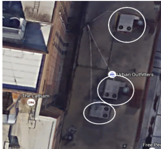
Figure 33: Aerial view of cooling equipment shaded by adjacent tall building
