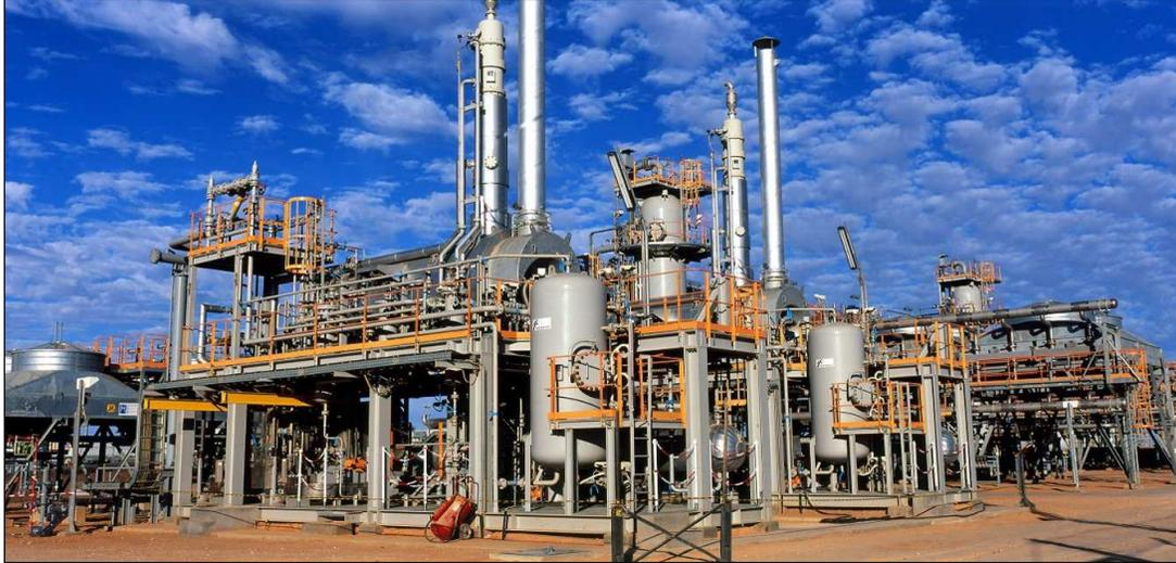
**Figure 1.2: An amine-based CO<sub>2</sub> capture system used to purify natural gas at British Petroleum's In Salah Plant in Algeria. Photo courtesy of IEA Greenhouse Gas Programme.**
