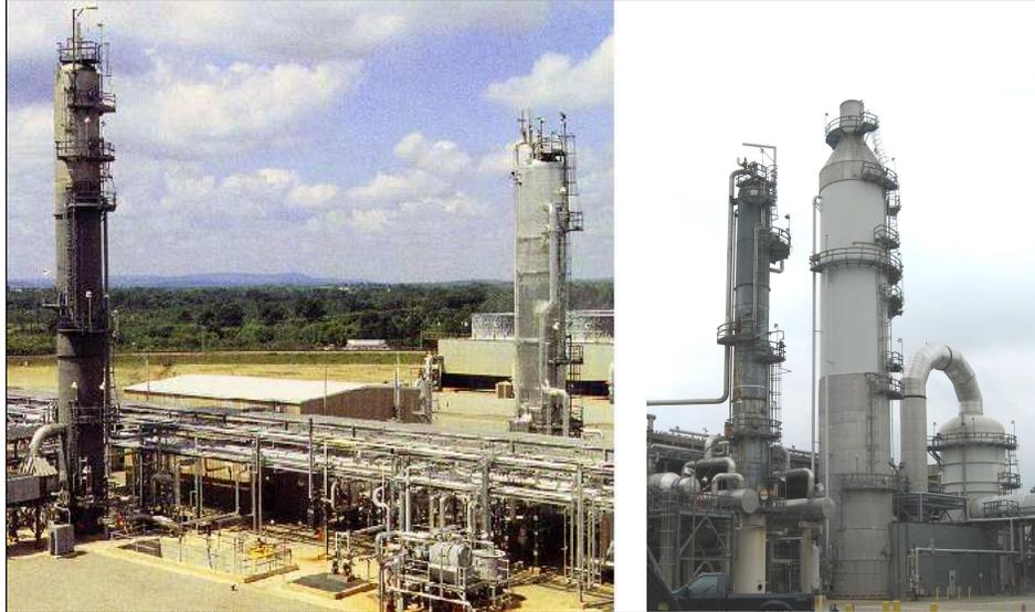
**Figure 1.3: Amine-based post-combustion CO<sub>2</sub> capture systems treating a portion of the flue gas from a coal-fired power plant in Oklahoma, USA (left) and a natural gas combined cycle (NGCC) plant in Massachusetts, USA (right). Photos courtesy of ABB Lummus, Fluor Daniels and Chevron.**
