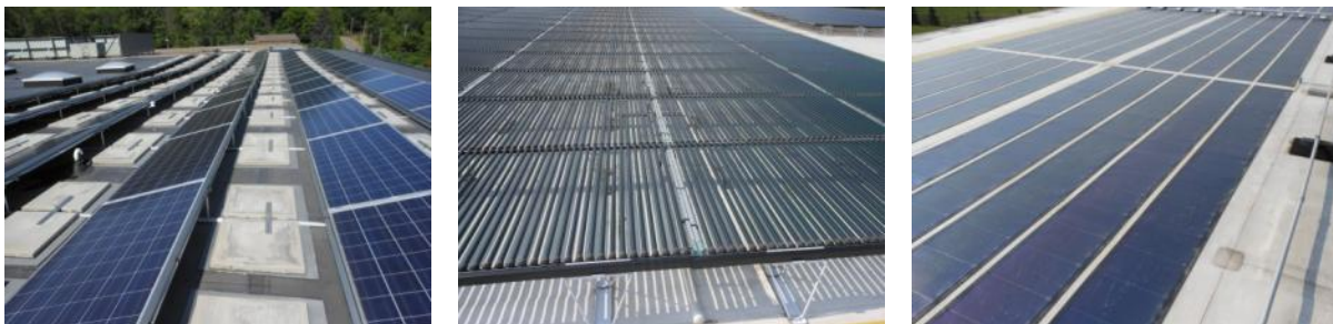
Figure 2-9: PV Panels types- ET Solar polycrystalline (left), Solyndra solar tubes (center), Unisolar thin film (right)
