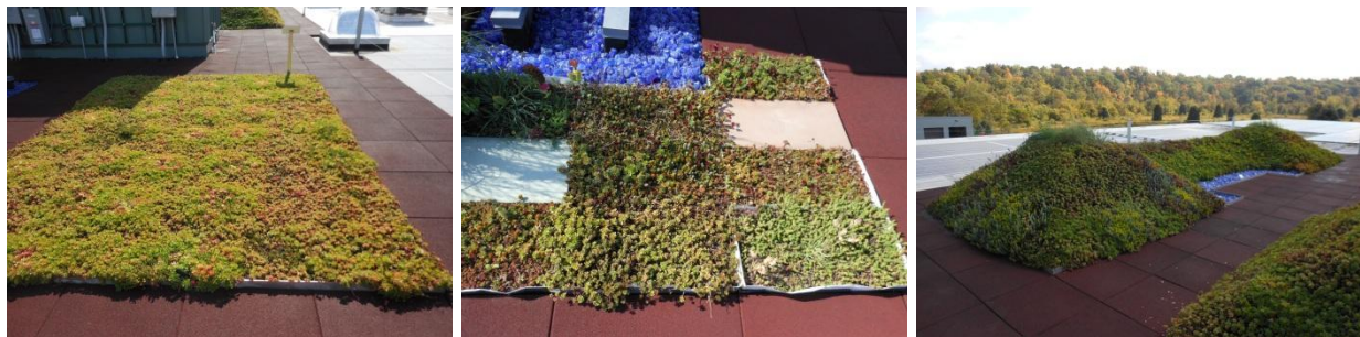
Figure 2-7: Images of small extensive green roofs: build up (left), modular (center), hilly (right)
