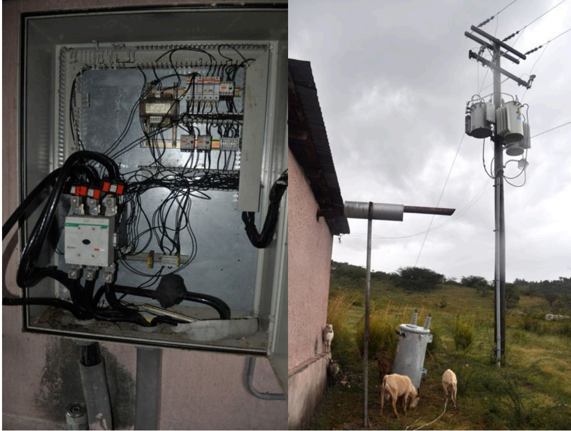
Figure B-4: The Port-a-Piment microgrid interconnection (L). The first distribution pole of the Port-a-Piment microgrid (R).
