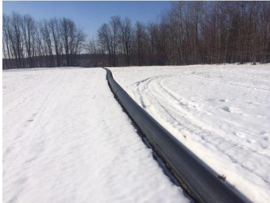
Figure 4.1: Water transportation through temporary piping.
