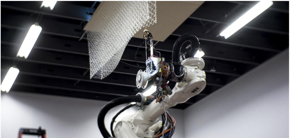
Figure 4. Ceiling retrofitting by FOAM process.
