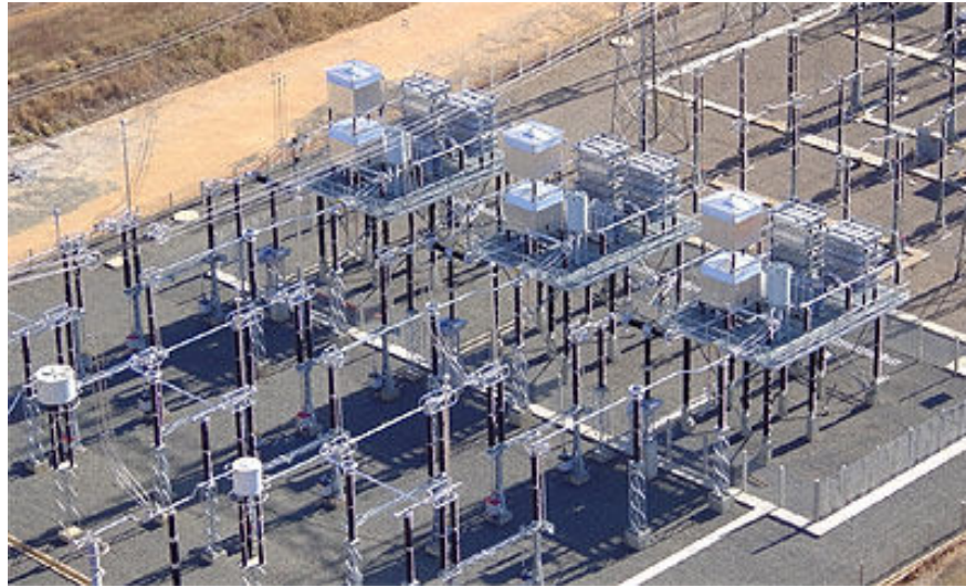
Figure 2.3: A thyristor controlled series compensator, a type of FACTS device, made by Siemens.
