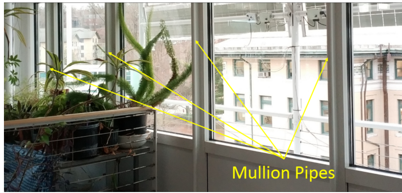
Figure 8.2: Hot Water Pipes Integrated on Window Mullions
