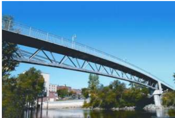
Figure 5.2. First UHPC engineering structure. A pedestrian bridge in Sherbrooke, Canada.
