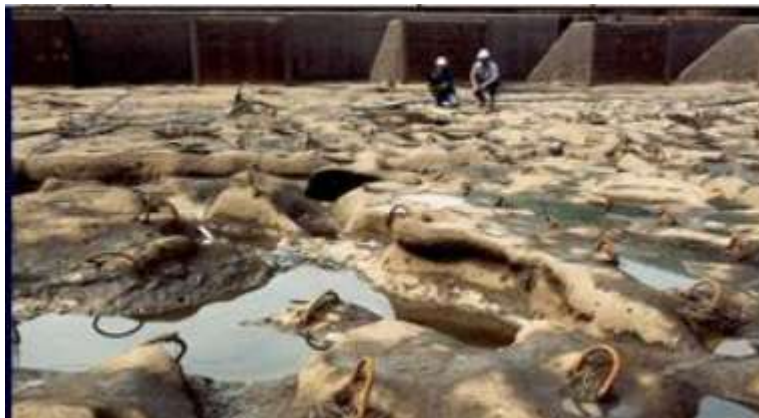
Figure 5.1. Eroded stilling basin of the Kinzua Dam in Warren County, Pennsylvania, in 1983.
