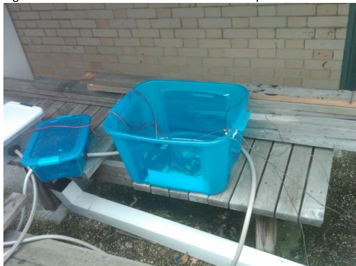
Figure 5.61 Weather tight control and pump boxes
