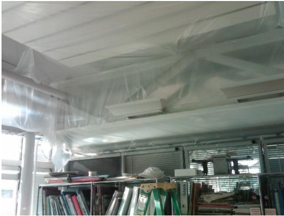
Figure 5.88 Enclosing the office space
