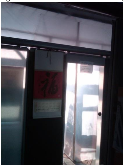
Figure 5.86 Plastic access doors
