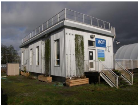
Figure 4.31 Installed wall-mounted trellis research panels (Connelly, Compton-Smith, Rousseau, & Huston, 2012, p. 26).
