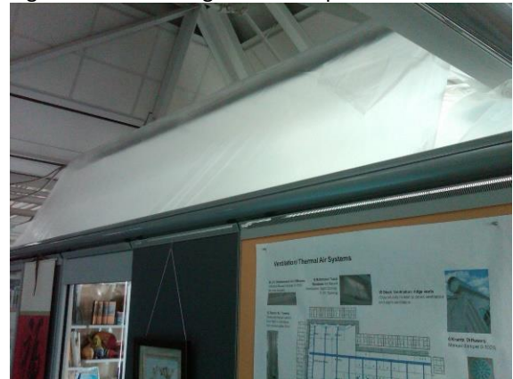
Figure 5.91 Plastic enclosure above partition
