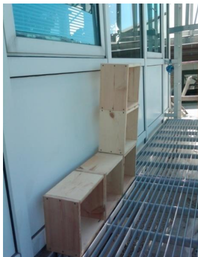
Figure 5.16 Empty Green Façade Planting Box Panels
