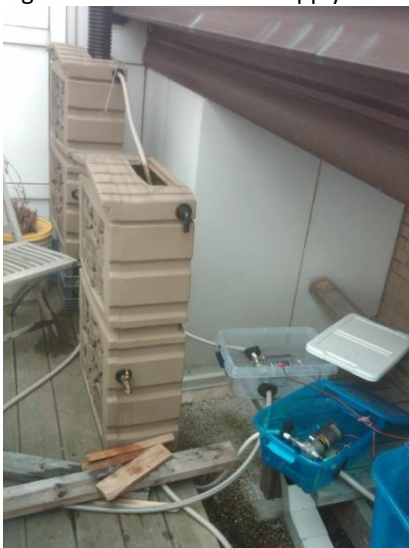
Figure 5.60 Irrigation pumps
