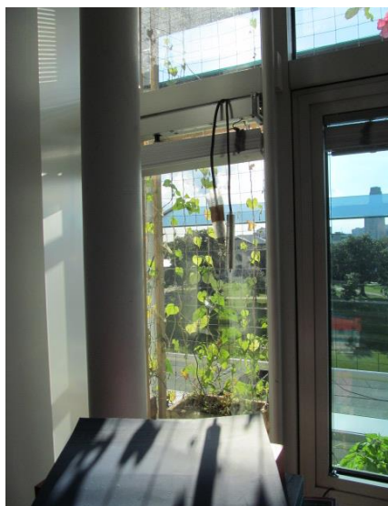
Figure 6.38 Fixed Glazed Panel Living Façade
