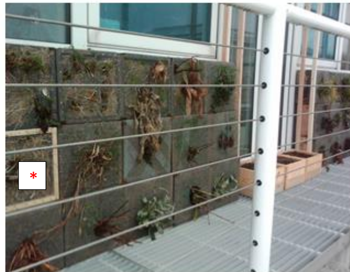
Figure 5.18 Photo images of Green Façade Wooden Panel Module construction and planting steps and façade installation.
