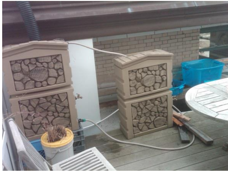
Figure 5.59 Two rain barrels with flexible downspout
