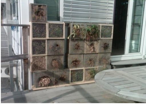
Figure 5.19 Planted panel installation on South Façade
